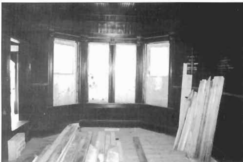
Reconstructing the Dr. George/Kemp dining room
